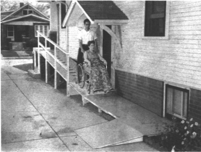
PLYWOOD PLATFORM IS LOWERED into position by rope to connect head of ramp with porch floor. Platform is stored on porch when ramp is not being used
