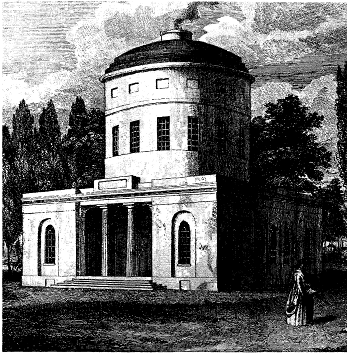
FIGURE FIVE: Latrobe's Water Works, Exterior View. The Water Works was built in 1800 and used until 1815; it was demolished in 1827-28. The building was faced in white marble, and became popularly known as "The Pepper Box." With dimensions of 60' x 60' x 60', it consisted of a round central pump room surrounded by offices. A harbinger of the Greek Revival in American architecture, the Water Works became, because of its location, the focus for civic occasions and public service. The engraving is from the Historical Society of Philadelphia.
