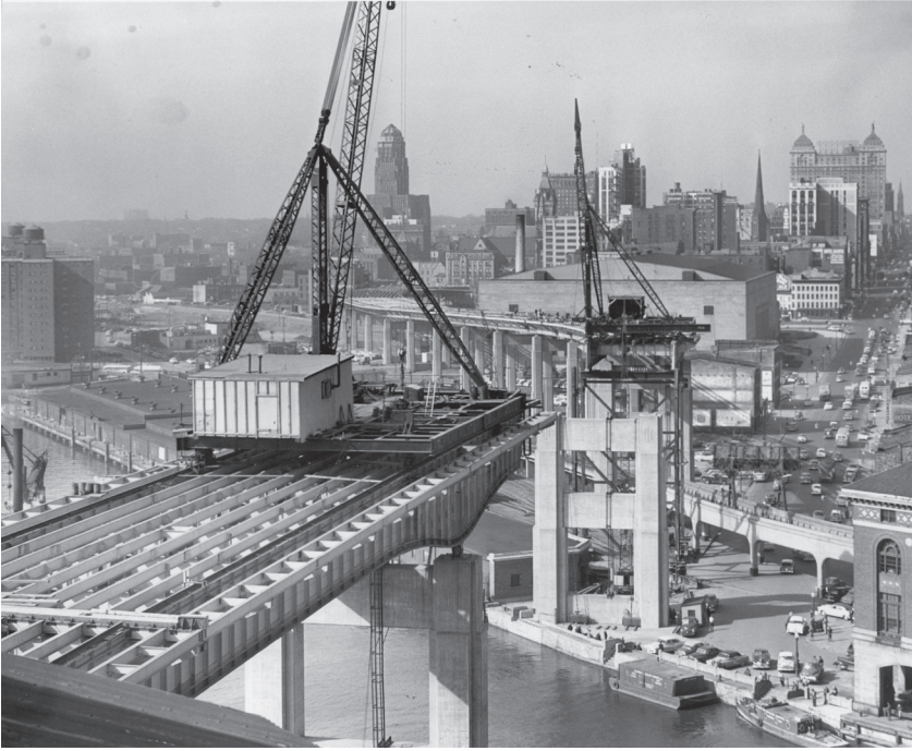
Figure 5: The Skyway under construction, April 14, 1955. Courtesy, Buffalo and Erie County Historical Society.
