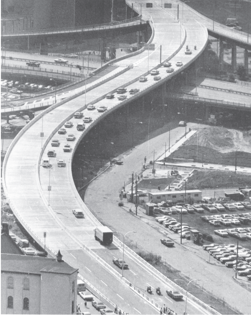
Figure 6: The renovated Skyway opens, 1976. Buffalo Courier Express Library Collection, Courtesy, E. H. Butler Library Archives, Buffalo State College.
