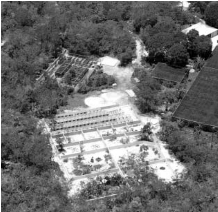
Aerial photo taken after completion of Team Blue's efforts. Photograph by John Binns.
