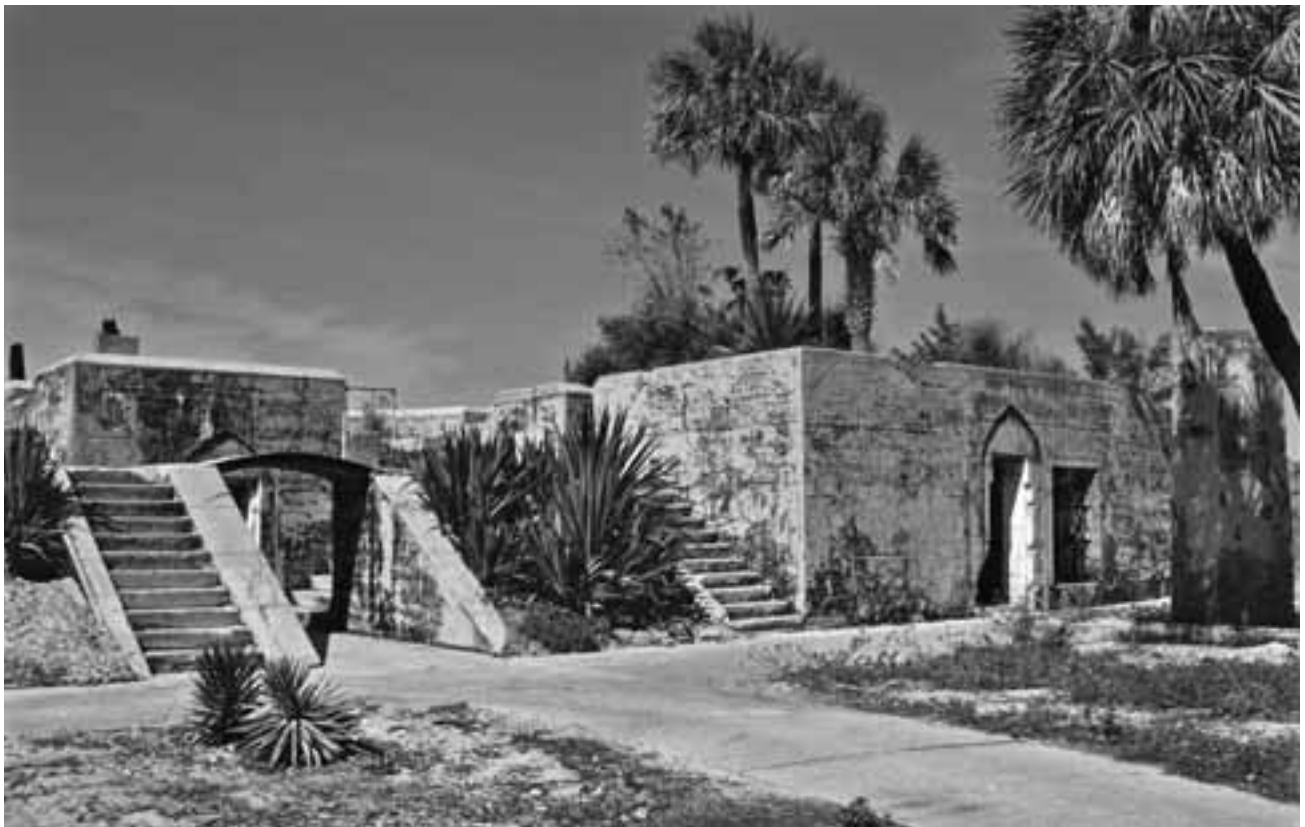
Mellon Battery at Fort Dade: Gopher Tortoises prefer the open areas afforded by the restoration of the buildings of the Spanish American-era fort.
