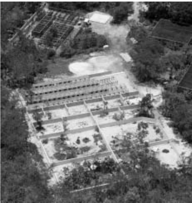
The Blue Iguana captive breeding and headstarting facility today. Beginning at the bottom of the photograph are four large adult breeding pens, four small adult breeding pens, and six adult holding pens. Next are 102 4 x 4 x 2 foot headstarting cages. The original fenced facility cages are in the upper left of the photograph.
