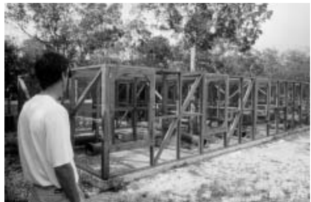
The first captive facility built in the Botanic Park shown at completion in 1996. The facility was funded by Milwaukee Country Zoo and its partner Foundation for Wildlife Conservation. The facility included 12 8 x 8 foot and 16 4 x 4 foot cages. Photographer unknown.
