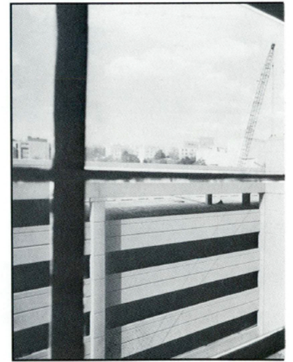
A northeast view of the new parking garage from a window in Allen Field House
