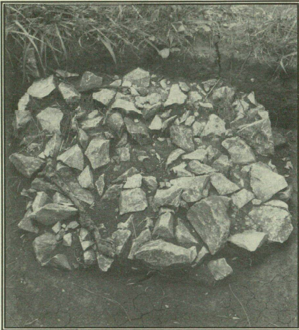
Figure 7. Photo of subfooting.
