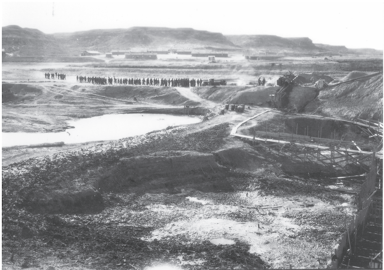
Figure 14. View of the dam under construction and the camp, view toward the west. (Courtesy of Larry Hoeme and the Scott County Historical Society)
