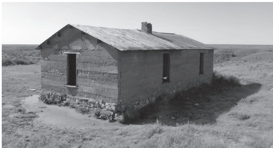
Figure 22. Cast concrete house, view to southwest.
