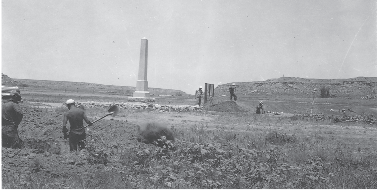
Figure 5. Wedel's 1939 excavation. In 1970 the monument was moved from the location shown in this photograph. (Courtesy of Nebraska State Historical Society, identification number 14SC1-20)
