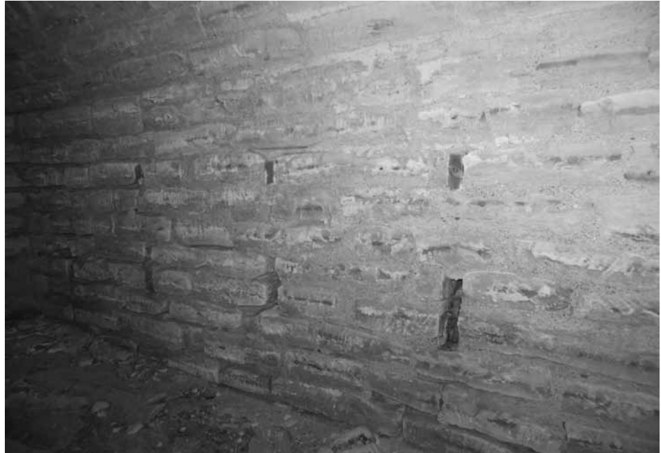
Figure 11. North wall view of Shimek cave 1, showing wooden blocks set in wall as shelf attachments.
