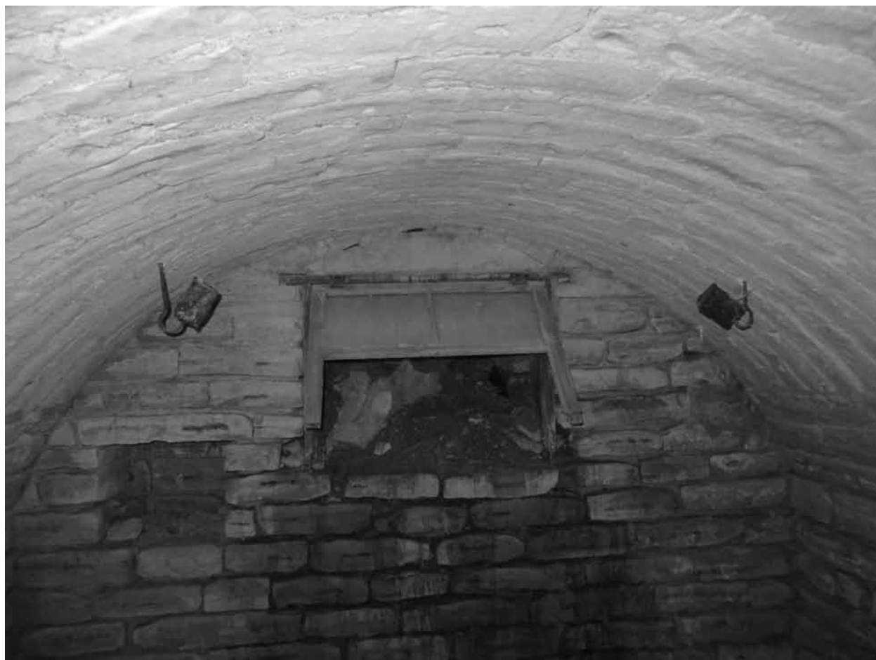
Figure 9. West end and ceiling view of Shimek cave 1, showing vent, niche, and hooks.
