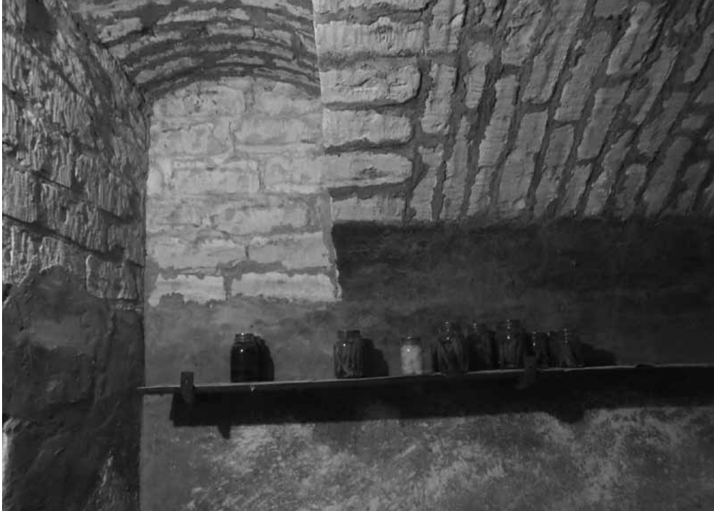
Figure 33. Interior ceiling view of Brown-Kusy cave, showing arch stone orientations and metal bar shelf supports.
