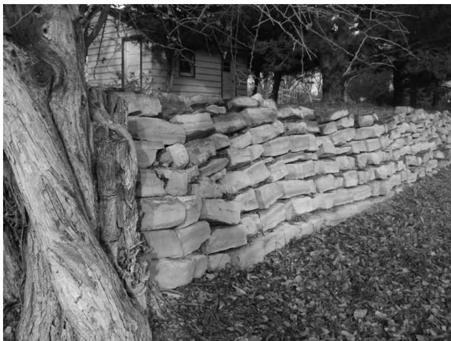
Figure 3. Retaining wall built with recycled Postrock limestone from Republic County area, Hebron, Nebraska.
