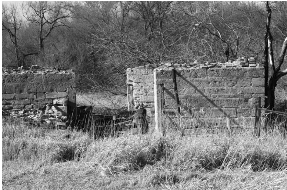
Figure 9a. Myers barn stone foundation, view northeast.
