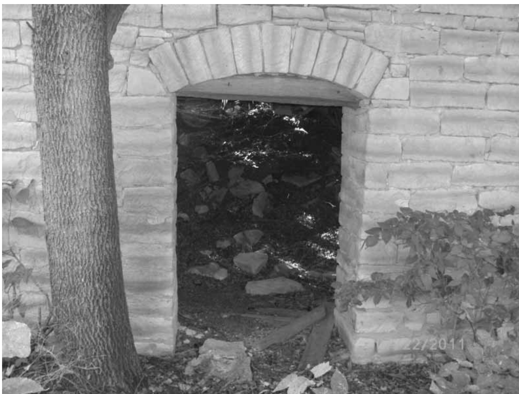
Figure 6a. Kiperta barn, view west, 2011.
