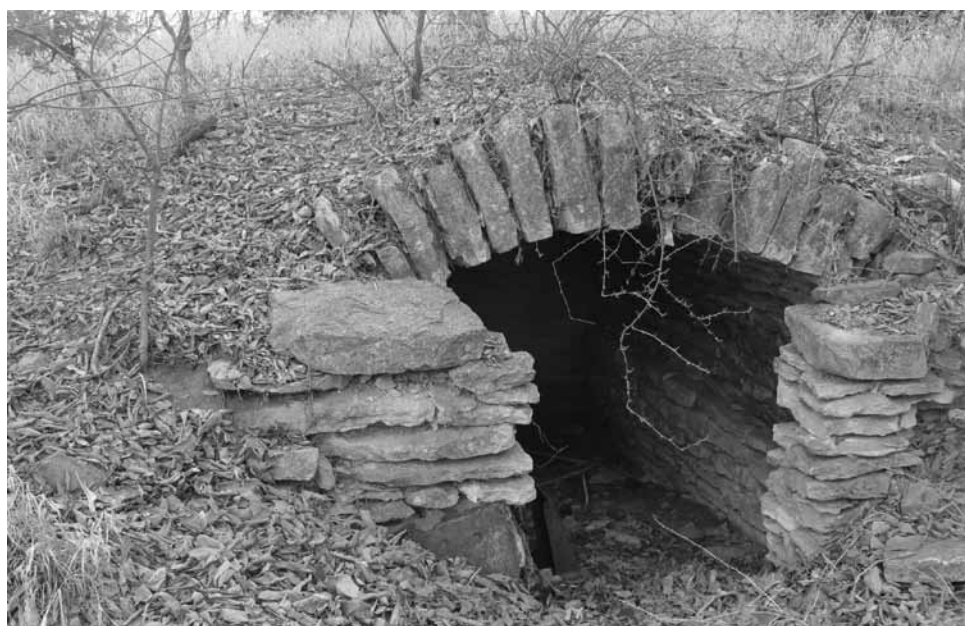
Figure 37b. Double-faced walls with rubble cores. East wall view of Wagner cave, showing double face.
