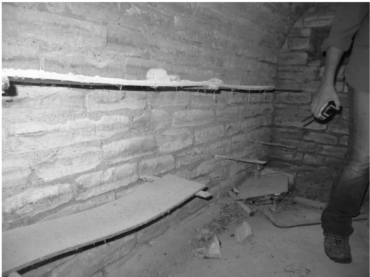
Figure 38. South wall view of Shimek cave 1, showing metal bars built into wall as shelf supports.
