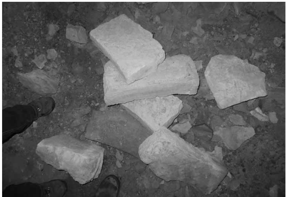
Figure 12. Collapsed arch stones of Shimek cave 2, showing concave edge of stones set perpendicular to long axis of arch.
