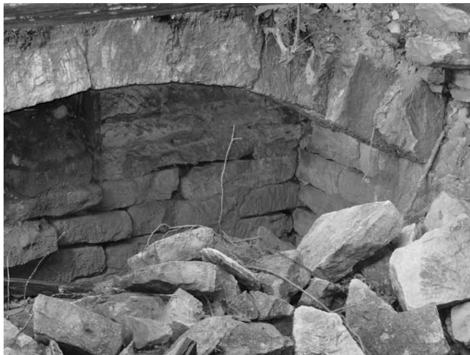
Figure 18. North end view of Kieffer 2 cave, showing north wall vent and remaining arch stones with tooled concave edges.
