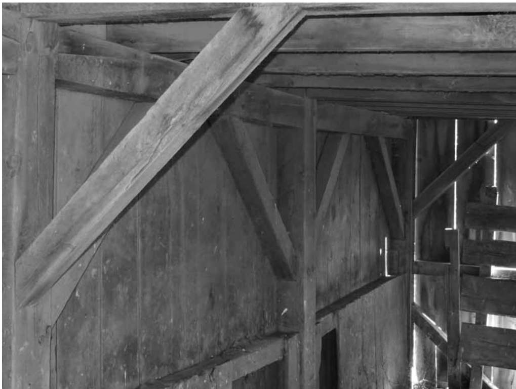
Figure 8b. Vakar barn interior view of timber frame construction.
