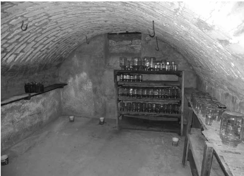
Figure 34. Ceiling and north wall views of Brown-Kusy cave, showing chute-type vent, metal bar shelf supports, and ceiling hooks.
