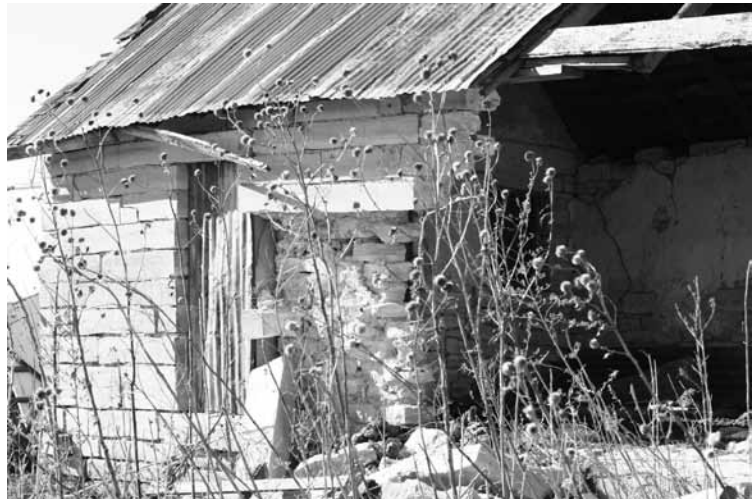
Figure 4c. Martin-Klima stone cabin, view southwest, 2012.
