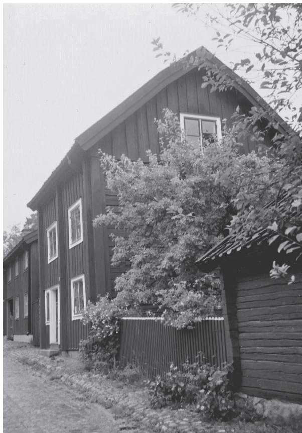
Figure 3. Red timber building in Linköping's Old Town, built by Mr. Andersson for his staff. Photograph © Lewis N. Ballantine.
