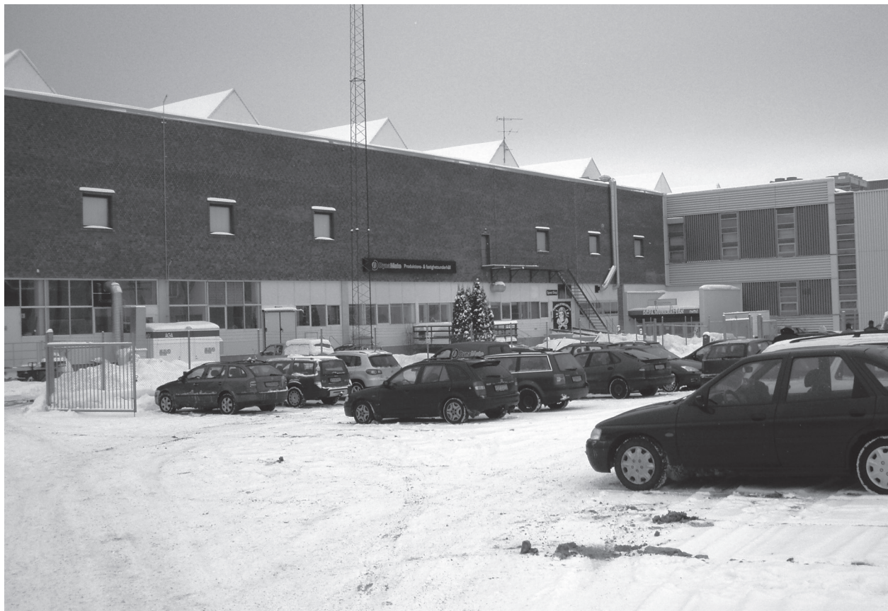
Figure 5. Stockholm City Council's storage facilities, Tumba, Sweden. Photograph © Lewis N Ballantine.
