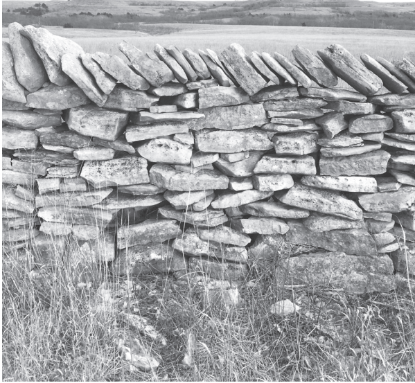
Figure 5. Wabaunsee County limestone fence associated with the Joseph Schutter homestead, archeological site number 14WB335. The oblique coping is typical of traditional Kentucky Bluegrass Region fences.
