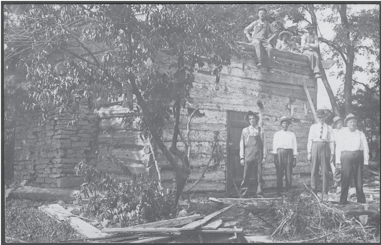
Figure 13. Dismantling cabin for move to park, 1911 or 1912. Courtesy of kansasmemory.org, Kansas Historical Society.
