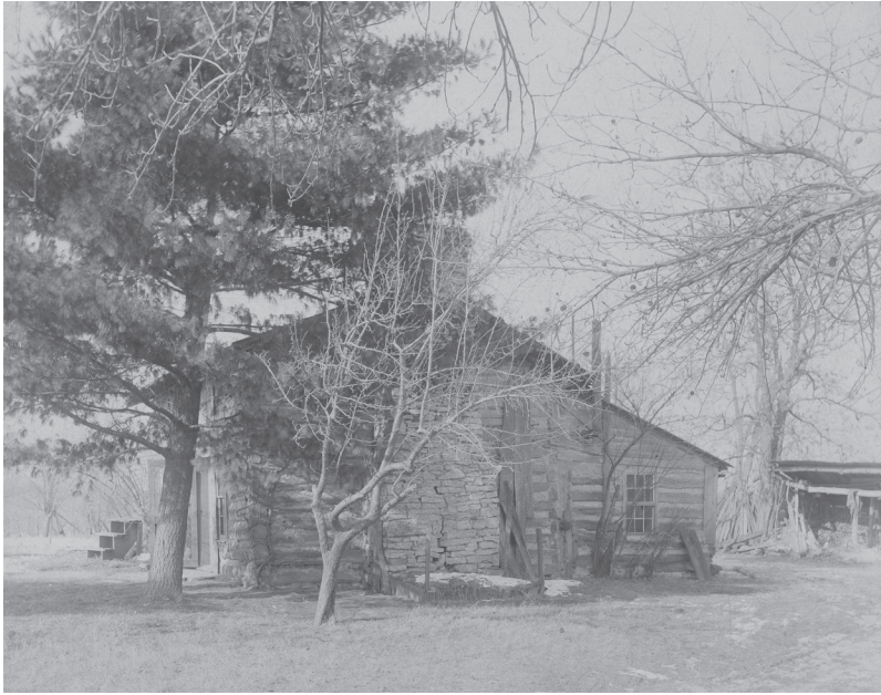
Figure 8. East side of the original cabin. The addition built by John Brown, his sons, his son-in-law, and Samuel Adair is the left half of the structure. Excavation units near the outbuilding in this image did not find evidence of it. Courtesy of kansasmemory.org , Kansas Historical Society.
