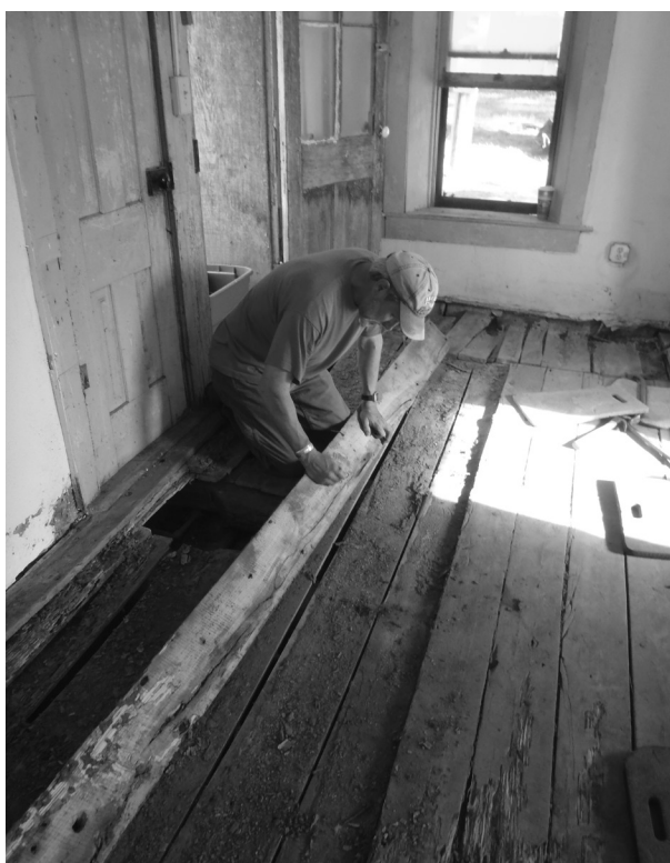
Figure 19. Chris Hord marking boards for later replacement.
