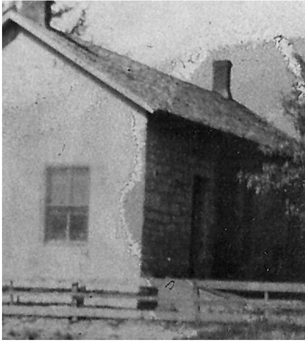
Figure 32. Detail showing the cellar door from a photograph taken prior to 1901.
