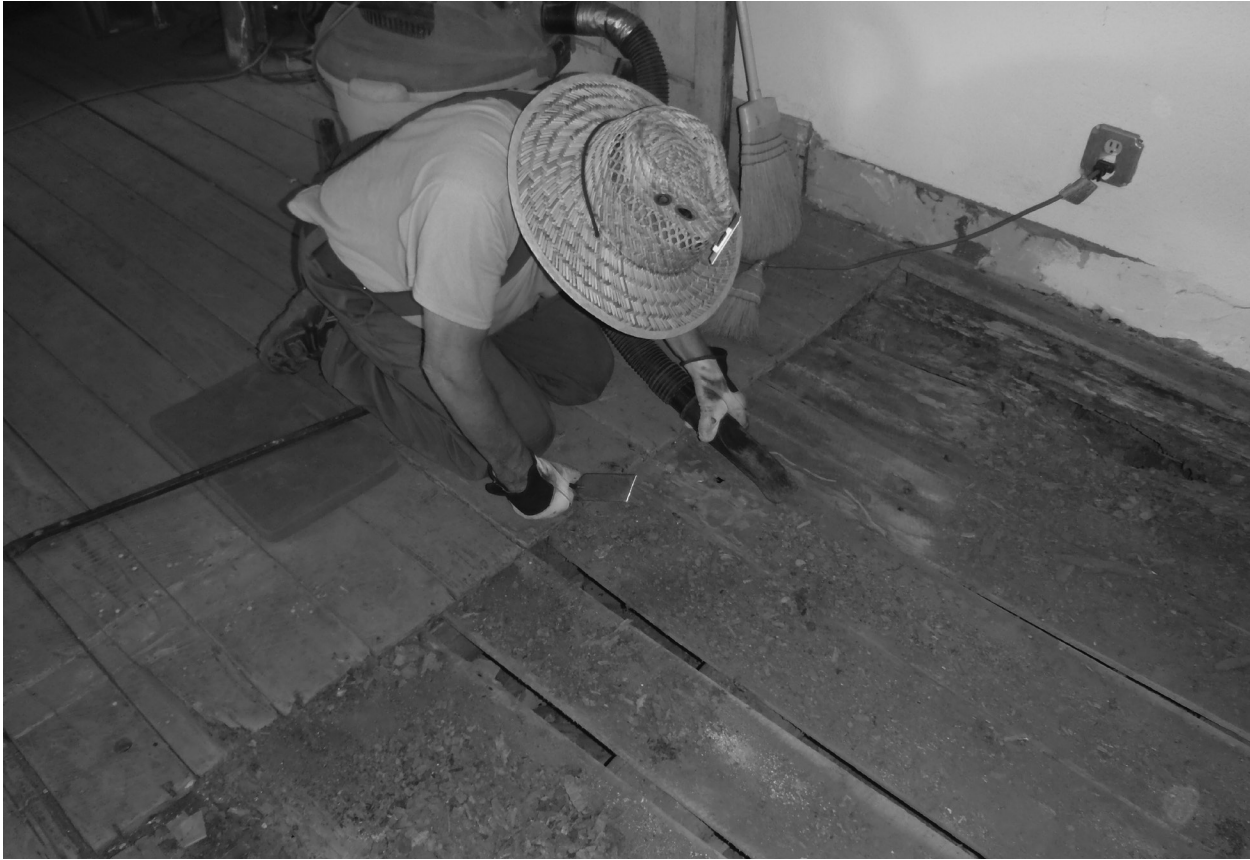
Figure 17. Lou Madden vacuuming up fill from between floorboards for screening.
