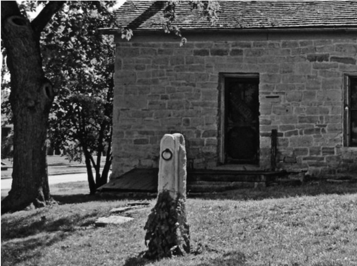
Figure 23. Limestone hitching post east of the building.
