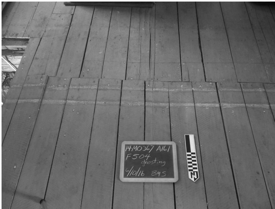
Figure 31. Ghost outline of former south interior wall.
