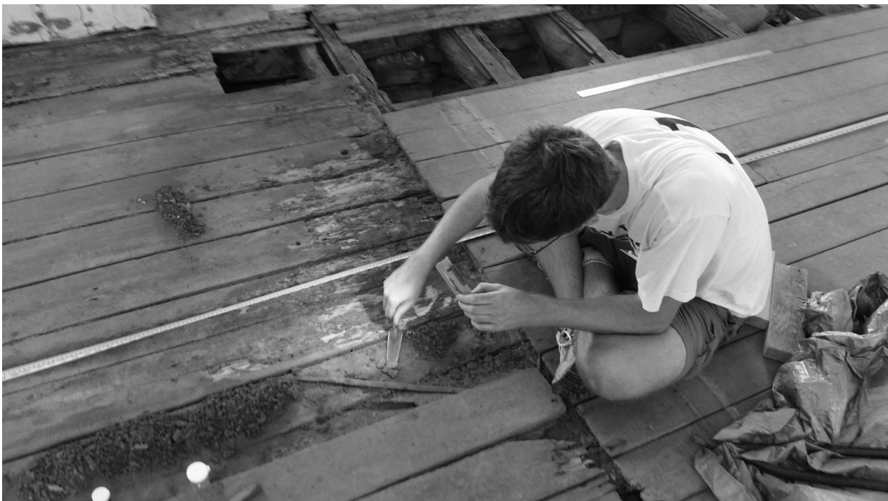
Figure 16. Neil Briggs excavating soil between floor boards.
