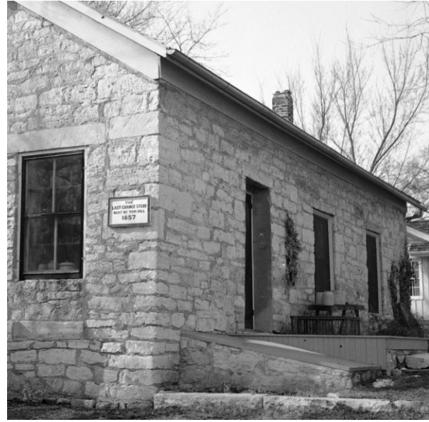
Figure 34. Detail of the cellar door and front porch from a photograph taken after 1990.
