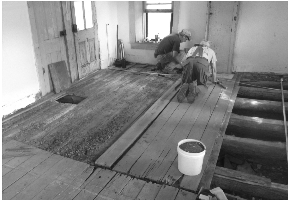
Figure 18. Boards in the N Center sector that were left in place.
