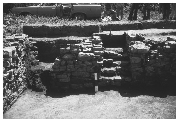
Figure 6. View of the south cellar wall, showing entrance and window locations.
