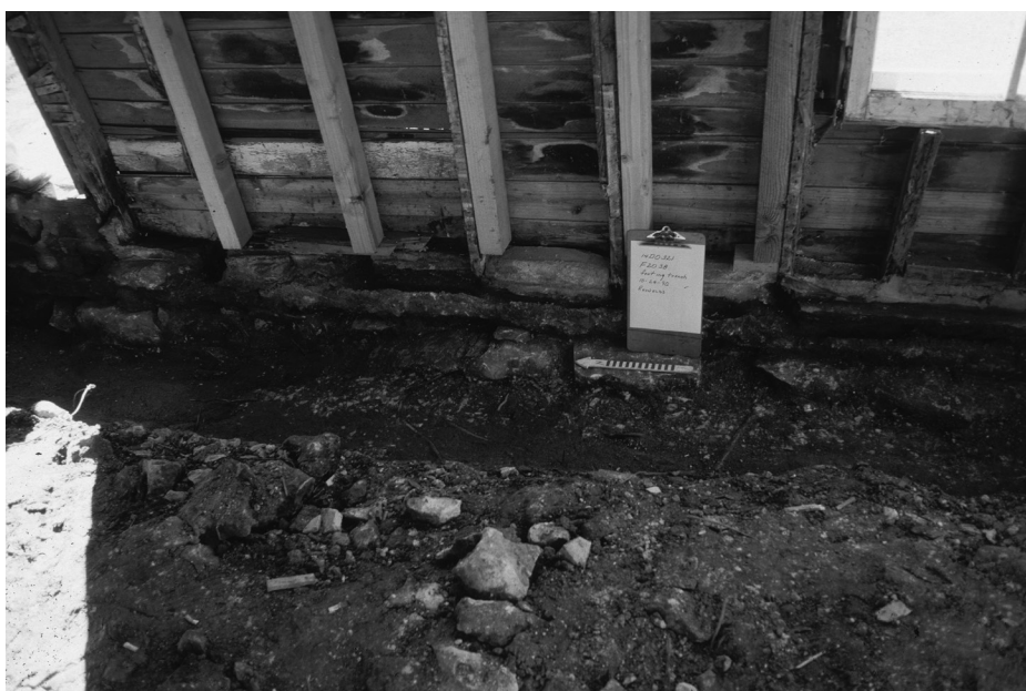
Figure 8. Builder's/ footing trench, exposed in 1990. North arrow is incorrect.
