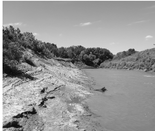
Figure 29. Exposed root end of a buried tree in the new channel of Stranger Creek in 2017. Photograph by Demaranville.
