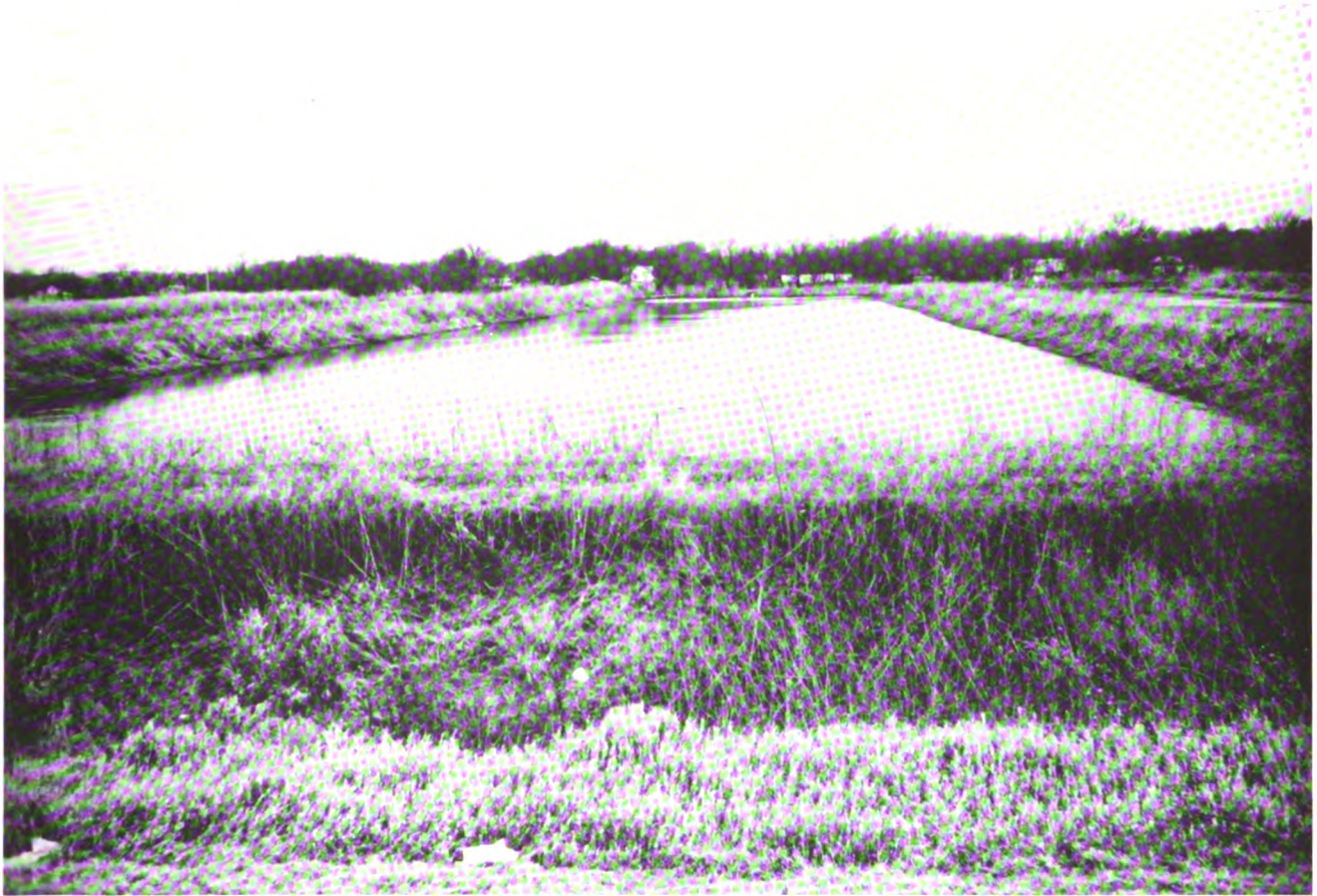
FIG. 16. View of community sewage lagoon. Large sewage lagoons can be easily constructed in soils with slight limitations, where the soils are nearly impermeable, are nearly level, lack coarse fragments, are not flooded, and have a good engineering classification for embankment construction and compaction. In some cases lagoons are the cheapest method of sewage treatment for communities; sewage lagoons can also be used for individual houses where soils are impermeable and where adequate land area is available.
