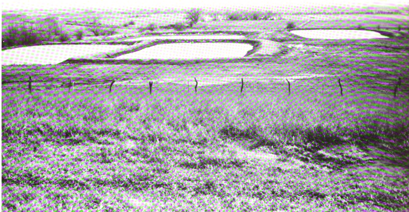
FIG. 17. View of lagoons on sloping soils. Soils with slopes greater than two percent have moderate limitations for sewage lagoons, because more earth must be moved than on slopes less than two percent. On slopes steeper than seven percent, sewage lagoons may not be feasible. Where large volumes of sewage are to be treated, several lagoons are generally built in series to handle wastes by stages—because certain holding periods are required for waste stabilization and oxidation.
