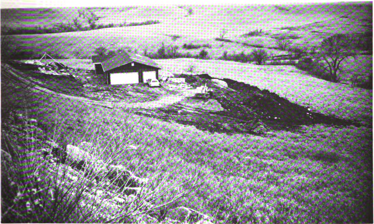
FIG. 14. Soils at this site have severe limitations for septic-tank seepage fields, due to slopes and slow permeability. Slope limitations have been improved with bulldozer grading, and the tile line for the seepage field has been placed in the looser fill below the house. With good engineering design and proper septic-tank maintenance, this sewage-disposal system could function satisfactorily, but pollution will be a hazard if the volume of soil material is not adequate for filtration.
