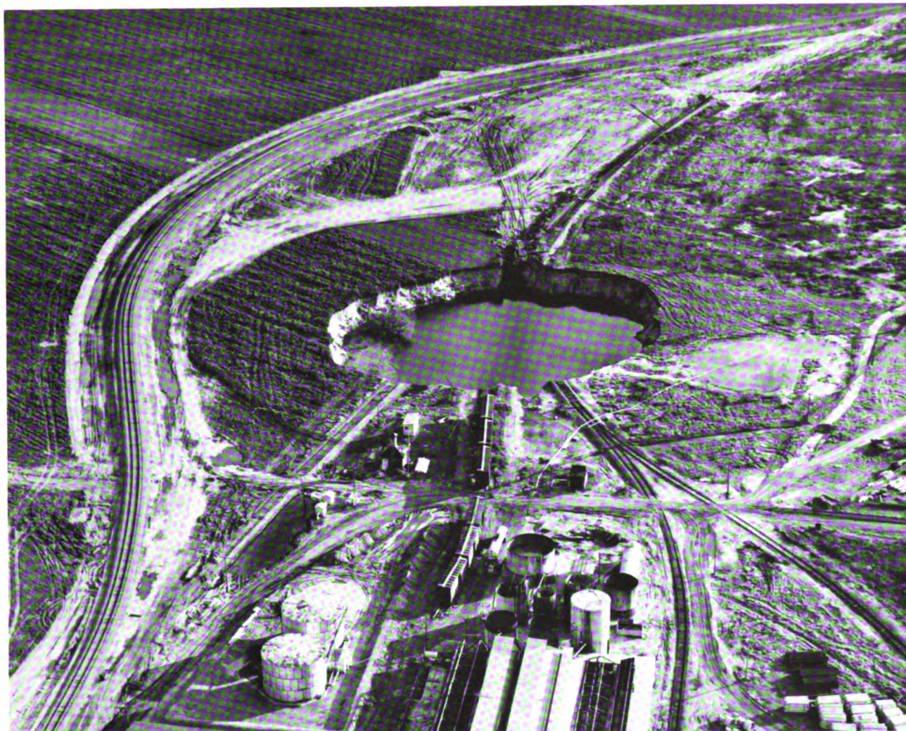
FIGURE 11.—Photograph by The Wichita Eagle and Beacon, November 12, 1974. Diameter of the stabilized sinkhole is 300 feet. View toward the south, with the Cargill salt processing plant in the foreground. Note that the tree mentioned in Figure 10 now stands in 18 feet of water within the crater near the east (left) bank. Missouri-Pacific railroad tracks have been relocated around the sinkhole.
