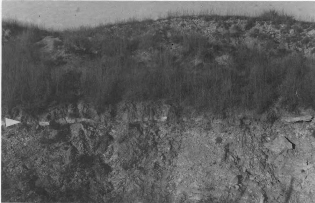
FIGURE 6—Smoky Hill chalk—Ogallala contact (arrow) in a roadcut in SESE sec. 34, T. 3 S., R. 17 W. Approximately 8.5 m (28 ft) of poorly cemented Ogallala overlies 8.9 m (29 ft) of chalk. The 10-cm-thick (4-in.-thick) chert bed at the top of the Smoky Hill Chalk Member is one of many in the member; these chert beds frequently occur at the top of the member because of their resistance to erosion. There is evidence that Paleo-Indians used this chert for the production of lithics (S. Holen, personal communication, 1990).
