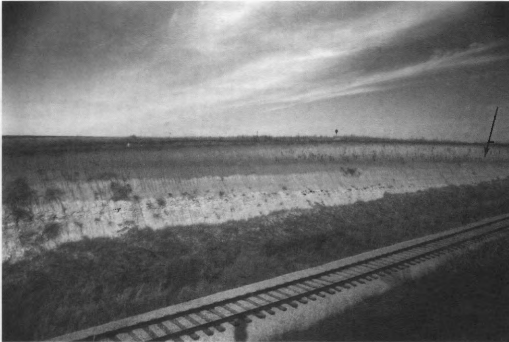
FIGURE 28—The Gilman Canyon Formation (arrow) exposed in the north face of a cut on the Missouri Pacific Railroad in NWNENE sec. 26, T. 4 S., R. 16 W. Peoria loess overlies the formation, and the Loveland Loess and Smoky Hill Chalk Member underlie it.
