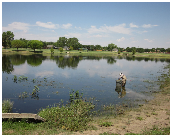
A lake located in a residential neighborhood in central Lubbock, Texas. The lake is part of the city's stormwater drainage project and is connected via overflow pipelines to other lakes in the drainage system. Note the impervious storm drains at the bottom left of the photograph.
