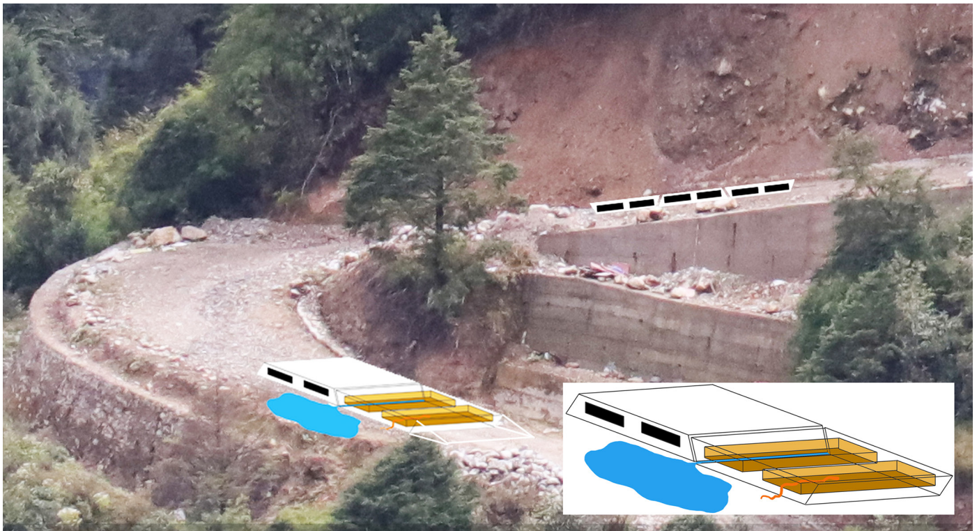
Figure 7. A second suggested mitigation measure to reduce the number of roadkilled Günther's Oriental Slender Snakes ( Trachischium guentheri ) is comprised of 60 cm-high hollow, trapezoidal concrete slabs laid in an alternate manner to allow for the passage of water and providing channels for snakes to pass.
