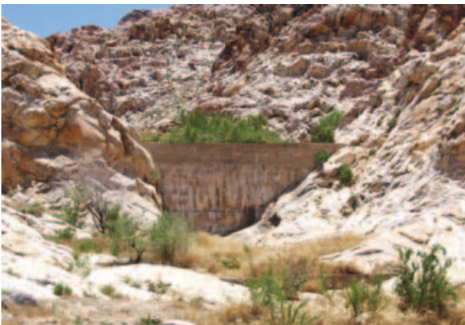
A large cement wall built by a cattle rancher named Warren Buffington in the early 1920s at the head of the canyon to retain water for year-round use.
