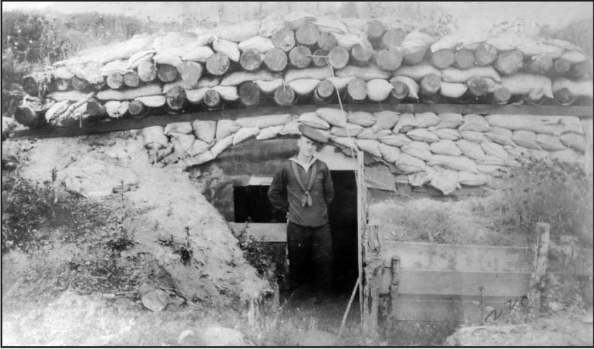
Fig. 3. “German Dugout (on Hindenburg Line),” Soissons, France, 1919. Photographer Unknown. Photograph 220, “U.S. Navy Treasures,” part of MSS 232. From the Collection of SCCHS.
