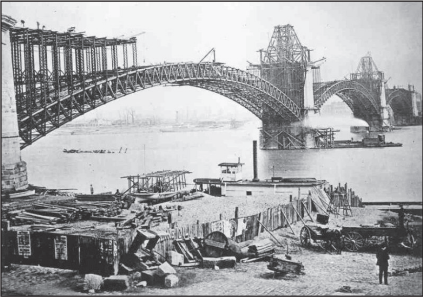
Fig. 16. Barton Bates joined his long-time friend James Eads in the effort to build a railroad bridge across the Mississippi River at St. Louis. Courtesy of stltoday.com
