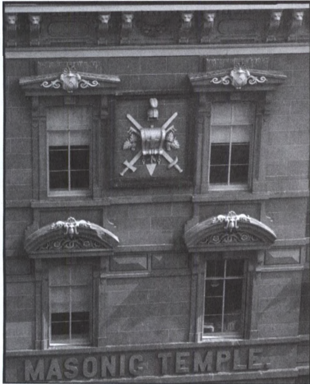
Fig. 11. Masonic Temple, detail of F Street façade, third and fourth floors, 2005. Cluss and Kammerhueber called for red brick construction for all of their buildings. The Masonic Temple differed only in that they specified sandstone facing for the two facades fronting on streets. Photograph by William Lebovich. Goethe-Institut, Washington, D.C.
