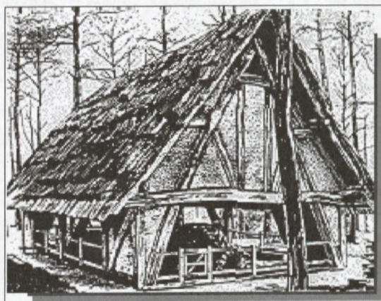
Fig. 3. Sketch of an earlier version of the simulated Jamestown Glasshouse before it fell victim to flames when its wooden shingles caught on fire. Courtesy of U.S. National Park Service
