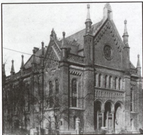
Fig. 8. Foundry Methodist Church (constructed 1863-64, demolished 1902). Located three blocks from the White House, Foundry Church was Cluss and Kammerhueber's first building located in the center of Washington and the first of his 1860s structures to be razed. Calvary Methodist Church, Washington, D.C.
