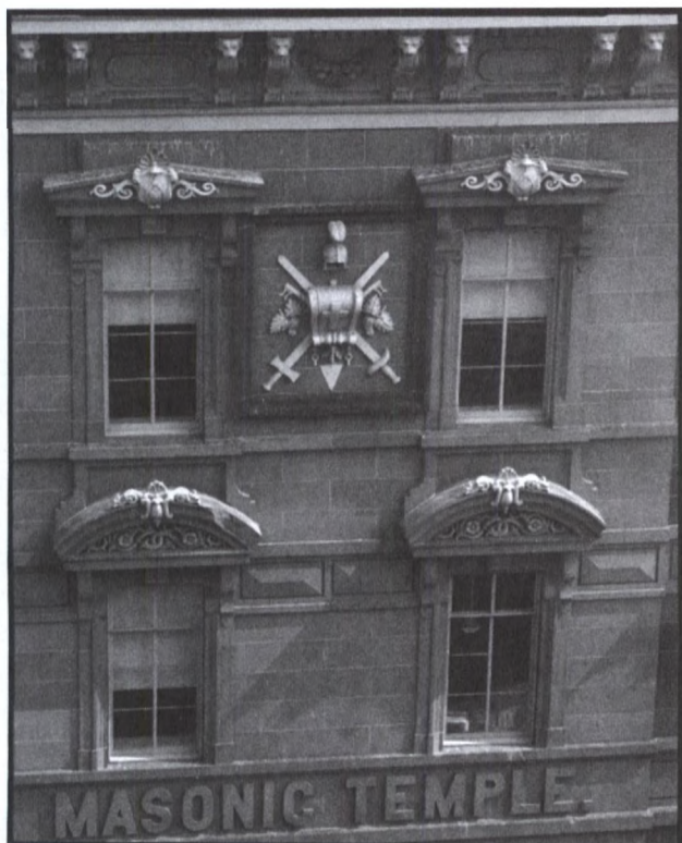
Fig. 11. Masonic Temple, detail of F Street façade, third and fourth floors, 2005. Cluss and Kammerhueber called for red brick construction for all of their buildings. The Masonic Temple differed only in that they specified sandstone facing for the two facades fronting on streets. Photograph by William Lebovich. Goethe-Institut, Washington, D.C.
